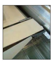
It is recommended that a short bead of silicone is applied over the connector cap gaskets at the points where the glazing bar capping seals make contact with them.
